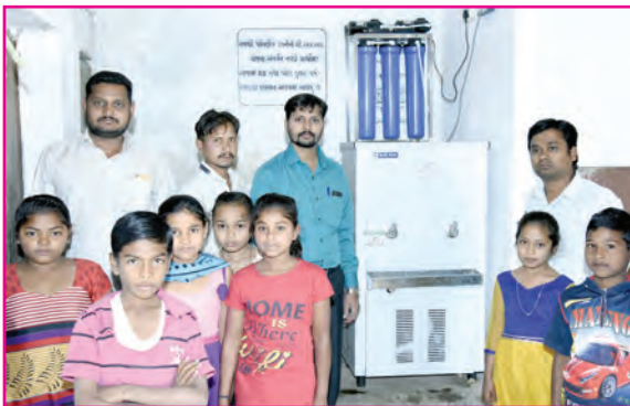
INSTALLATION OF WATER COOLER
